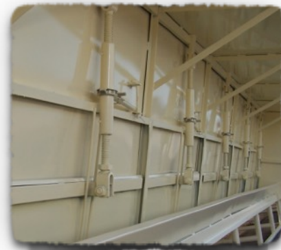
FEED FLOW DOOR LIFT ASSIST
